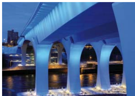
Bridge / Road Infrastructure lighting
